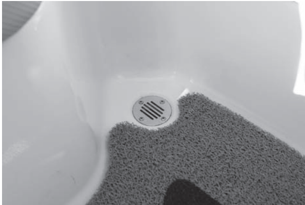
Figure B39: Liner Drain
