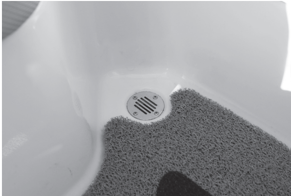
Figure B39: Liner Drain
